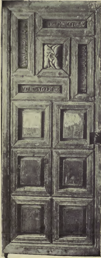
ONE OF THE ENTRANCE DOORS OF EL SANTUARIO, AT CHIMAYO, N. MEX.
